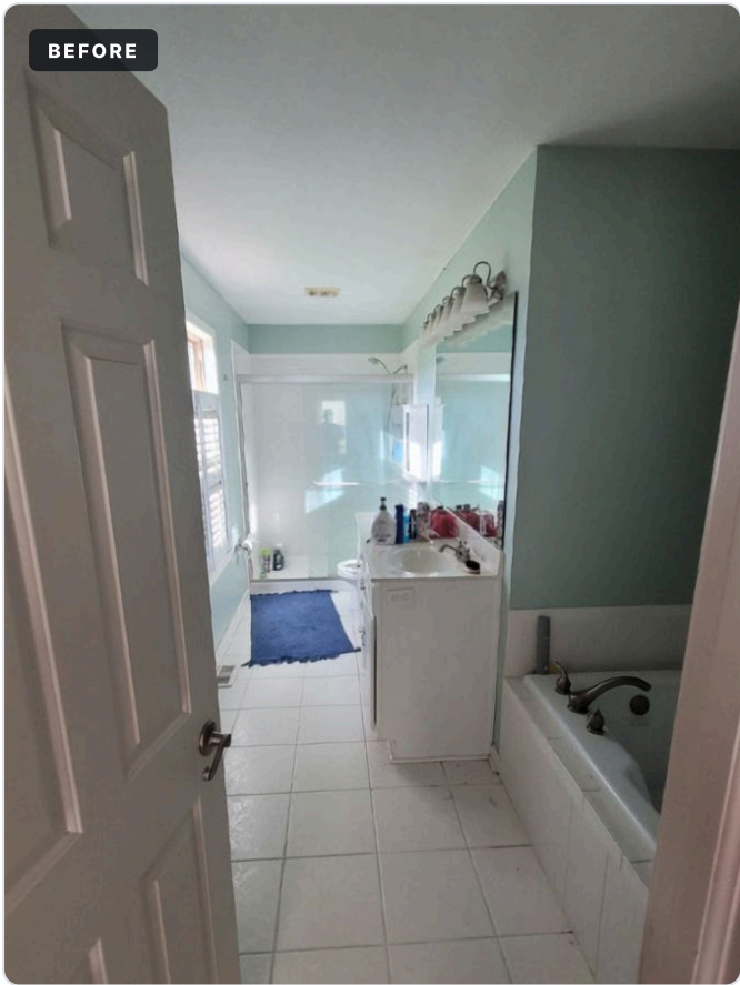
Before Primary bath Pre-existing Mar 3, 2026 · 9:26 AM
